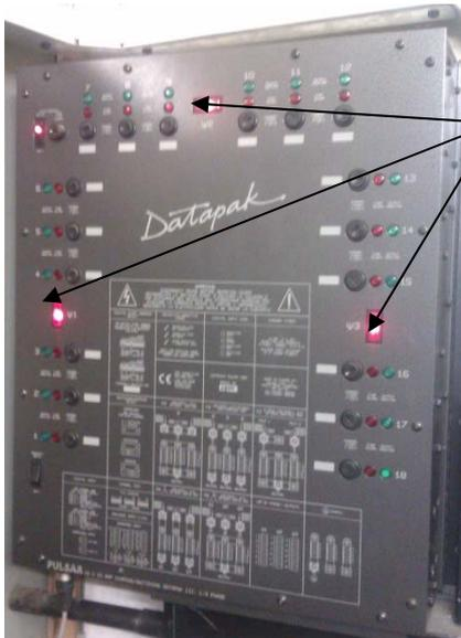
You can check that the dimmer pack is fully powered up by looking for the red lights on the front panel of the dimmer pack.
