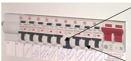
Switch 6 (from the left) controls the 32A supply for the Strand dimmer rack and may be down (off) if the dimmer is not being used. If the dimmer pack is required push this switch up to the on position.
